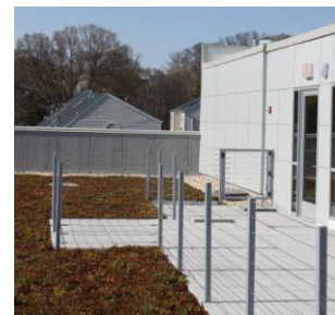
Macedonian's green roof
